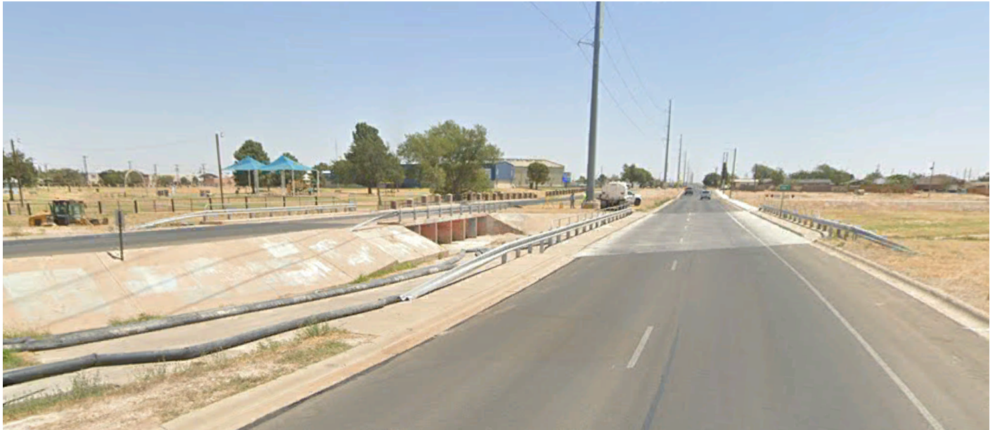
Photograph 2 - Existing Conditions of Scharbauer Drive at Midland Draw
